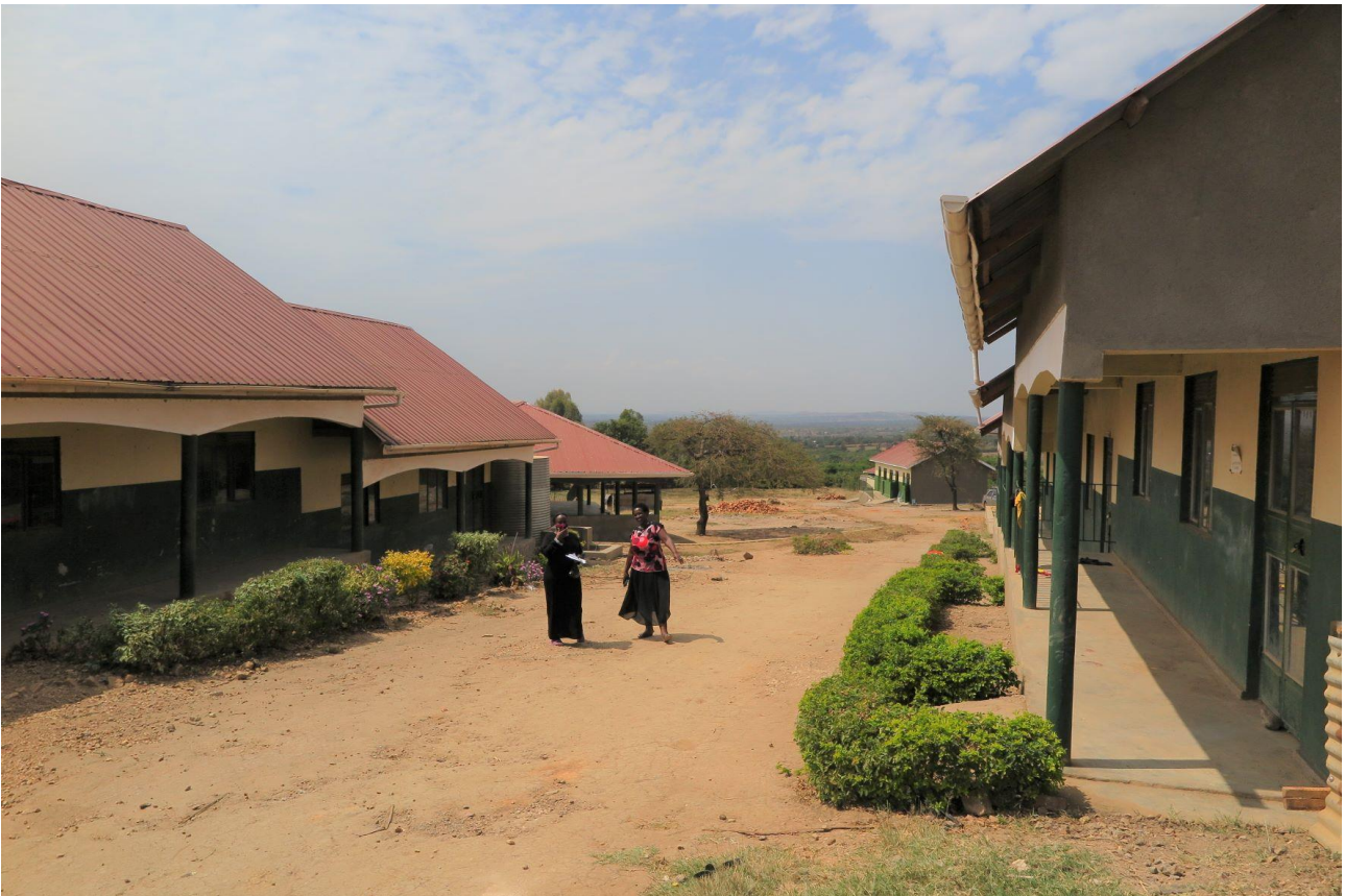
Left the classrooms of the Action Plan 2018 with at the end the Dining Hall (constructed this year). At the right the Nursery block of the Action Plan 2019 with in the back the Boys Dormitory, just built recently In the middle Madam Josephine from KACHICA Management, teacher and Chairlady of the Women group with Rachel Tushabe of Tusaidiane.
